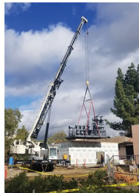
Heat exchanger placed in temporary building.
