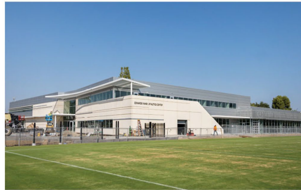
Edwards Family Athletics Center construction.
