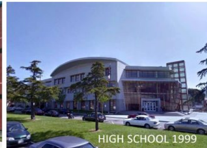
AUSD Existing School Facilities
